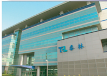
Hsinchu Industrial Park - ThaiLin
